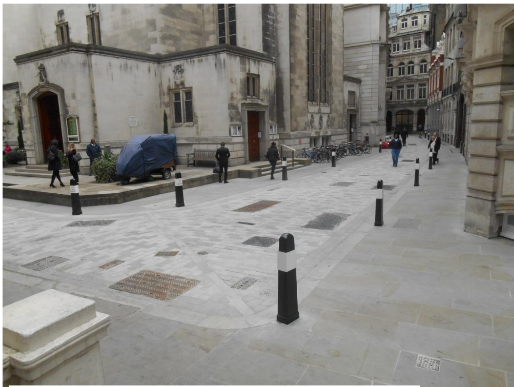
Austin Friars Central Section – After works
